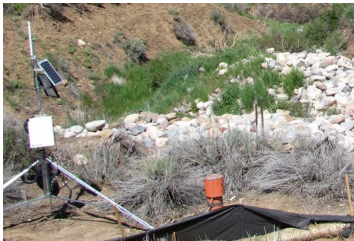
Telemetry equipment used to relay data to the Department of Energy from a well at the Durango Disposal Site.
