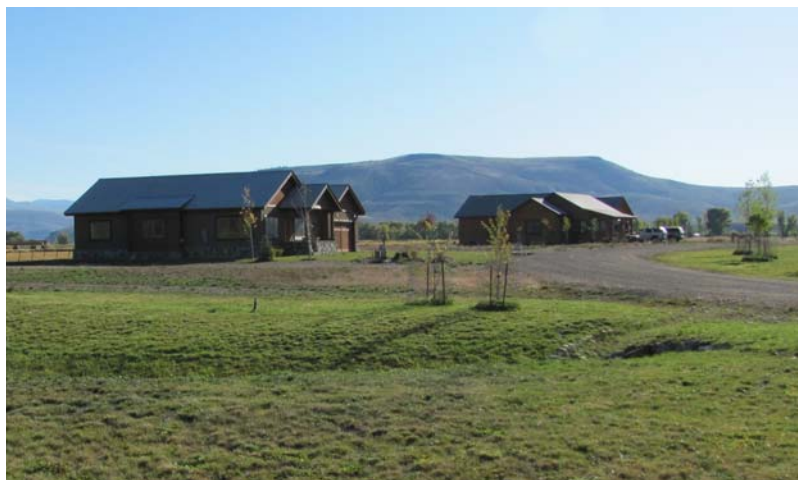
New homes constructed over the groundwater contaminant plume in Gunnison that are provided potable water from the DOE-State funded public water system.
