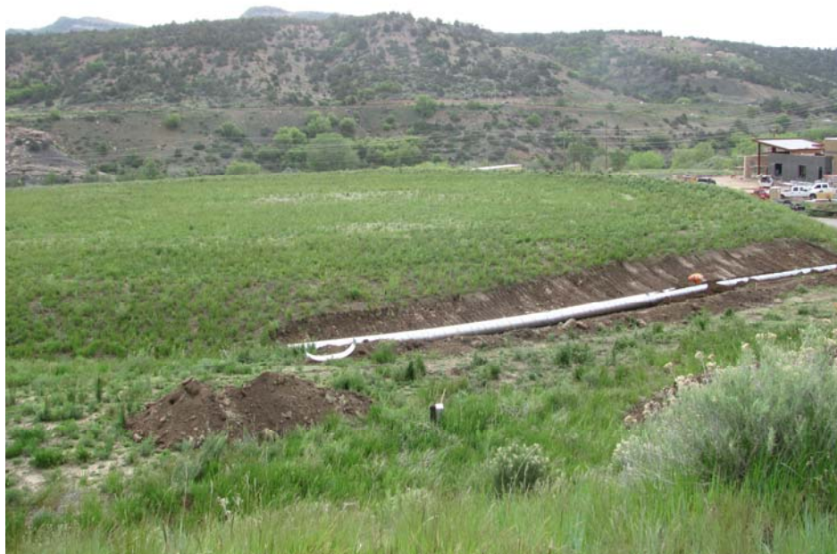
Durango Youth Baseball secured a long-term lease from the land owner, the Animas La Plata Water Conservancy District, to construct baseball fields on the property. Site preparation work is under way.
