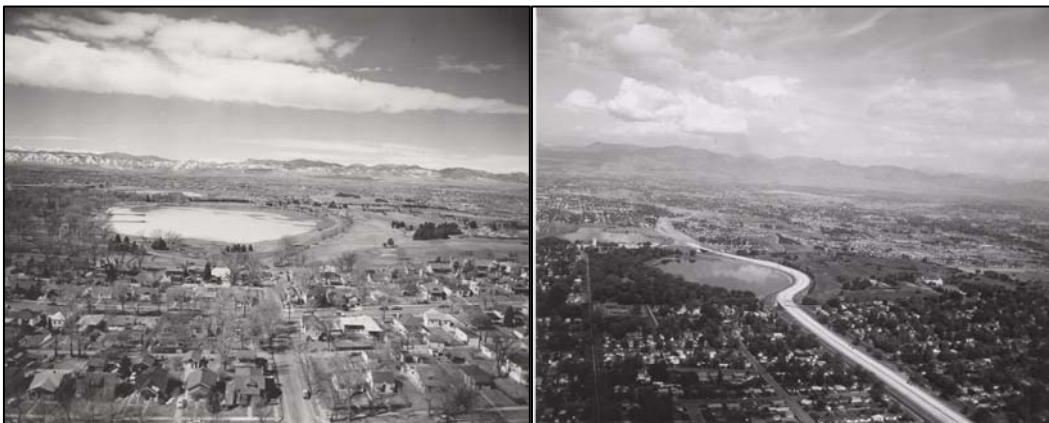
The Berkeley neighborhood and Berkeley Lake before and after the construction of I-70. Credit: CDOT Photo Archive
