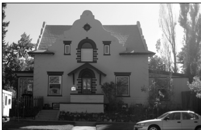
The West Washington Park survey area features a number of residential architectural styles and building types, including Late Victorian, Bungalow, Craftsman, and this relatively rare (for the area) Mission Revival. Photo by Marcy Cameron.
