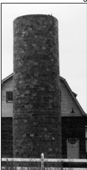
Curved block HCT silo at Shannon Farm in Lafayette (5BL.7260)
