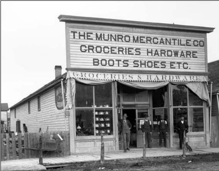
*George R. Porter's general store in Sneffels employs a false front to give the impression the one and one-half story building is actually a full two stories in height. The facade is of horizontal siding while the side wall is of vertical board-and-batten construction. The facade cornice is embellished with brackets.*
