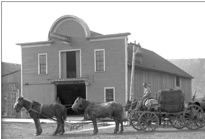
*This livery stable in Rifle is also a one and one-half story false front. Instead of a flat parapet, a semicircular pediment hides the upper gable end. Triangular peaked parapets are another common variation.*
