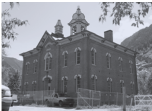
The Georgetown School, and restoration project leader Cindy Neely
