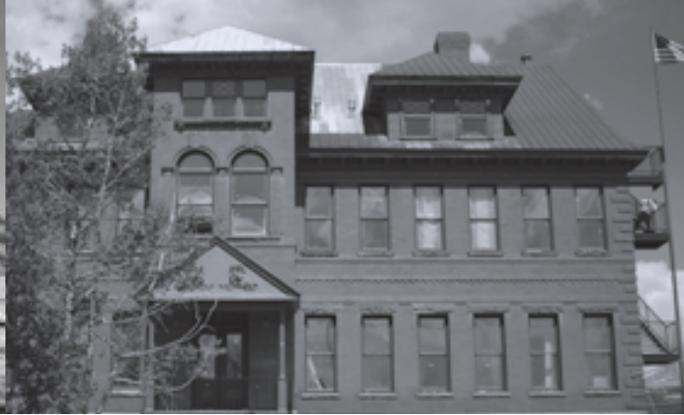
Saint Vincent's Hospital in Leadville after roof restoration
