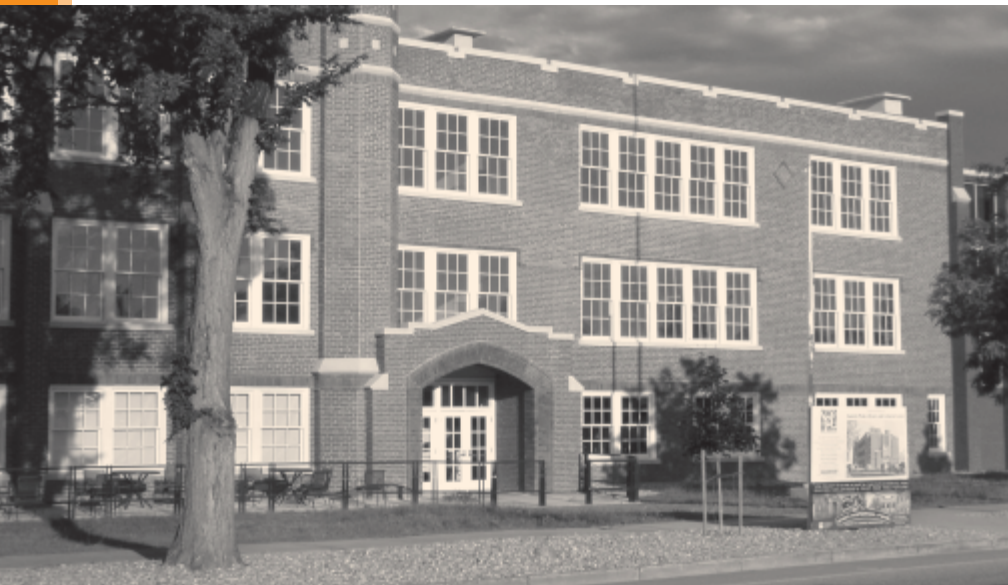
The new home of the Spanish Peaks Library (the former Huerfano County High School/Walsenburg Middle School) before (above) and after its exterior stabilization, masonry restoration, and replication of its historic wood windows.
