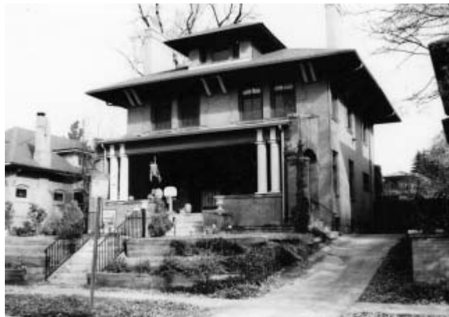
The John and Elivera Doud house in Denver, childhood home of Mamie Eisenhower
