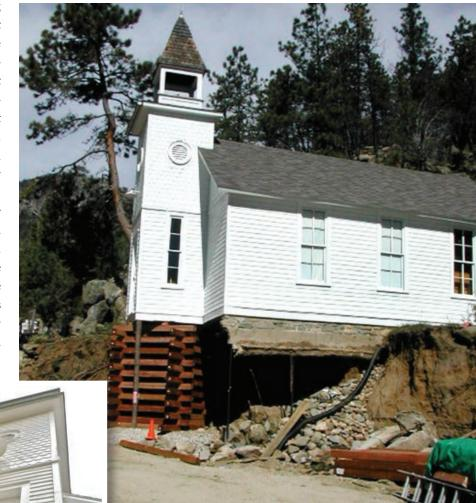
This page and facing: State Historical Fund emergency dollars enabled stabilization of Salina's historic Little Church in the Pines after floodwaters ripped away half the foundation.
