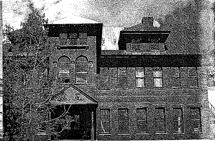
Saint Vincent's Hospital in Leadville after roof restoration
