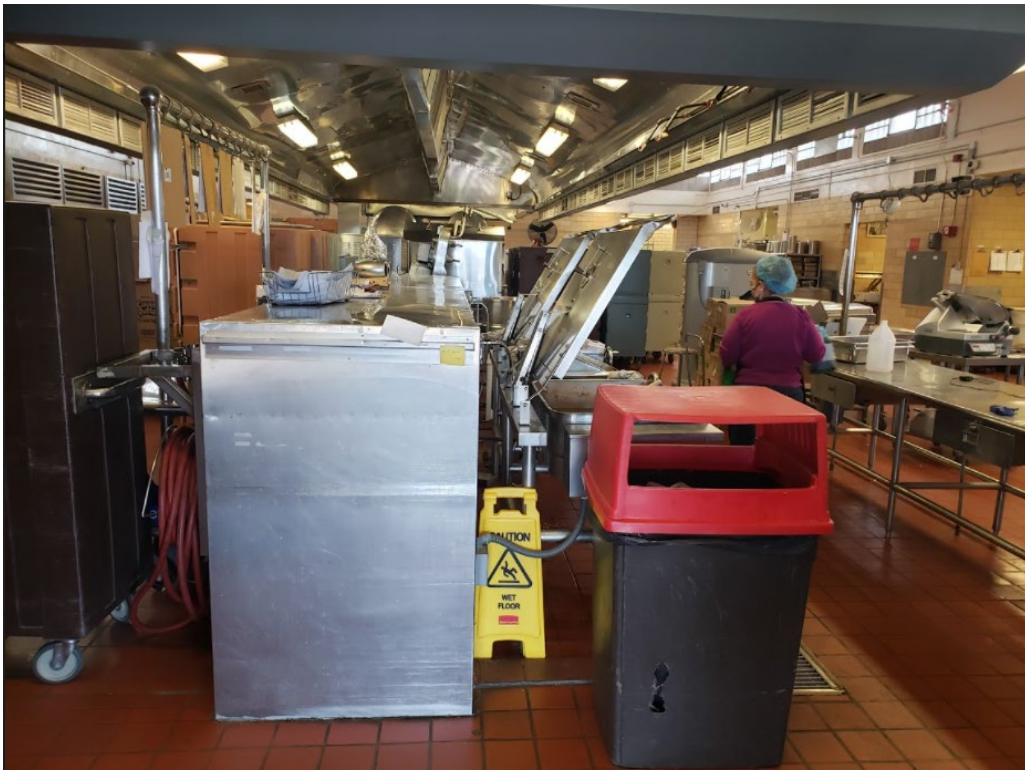
Current conditions within the CMHIP Kitchen, Bldg. 117
