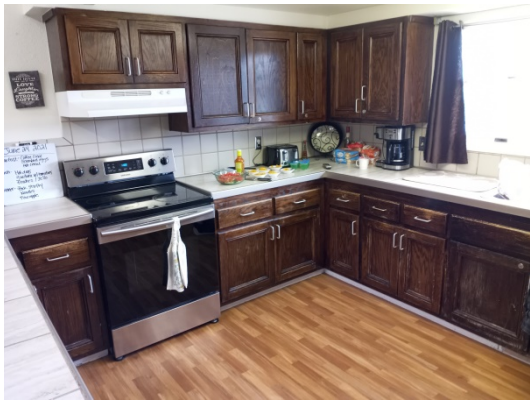
Outdated Kitchen with deteriorated cabinetry
