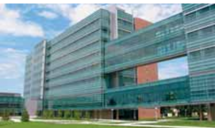
The University of Colorado at Denver and Health Sciences Center's Research Complex 1 at Fitzsimons
