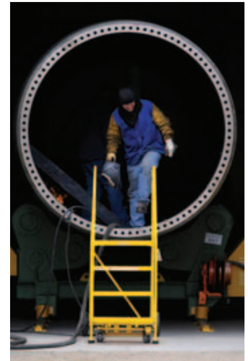
A worker climbs out of a large wind tower at the new Vestas plant in Pueblo.
