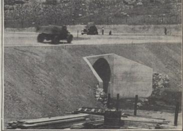
Metal plates in the arch are similar to those used in large culverts under highways and railroads. They have proved to be exceptionally strong and long lasting as they are heavily galvanized. Several of these multiplate, arches were used in numerous bridges constructed on state highway No. 12, west of Trinidad, by the Works Progress Administration.
