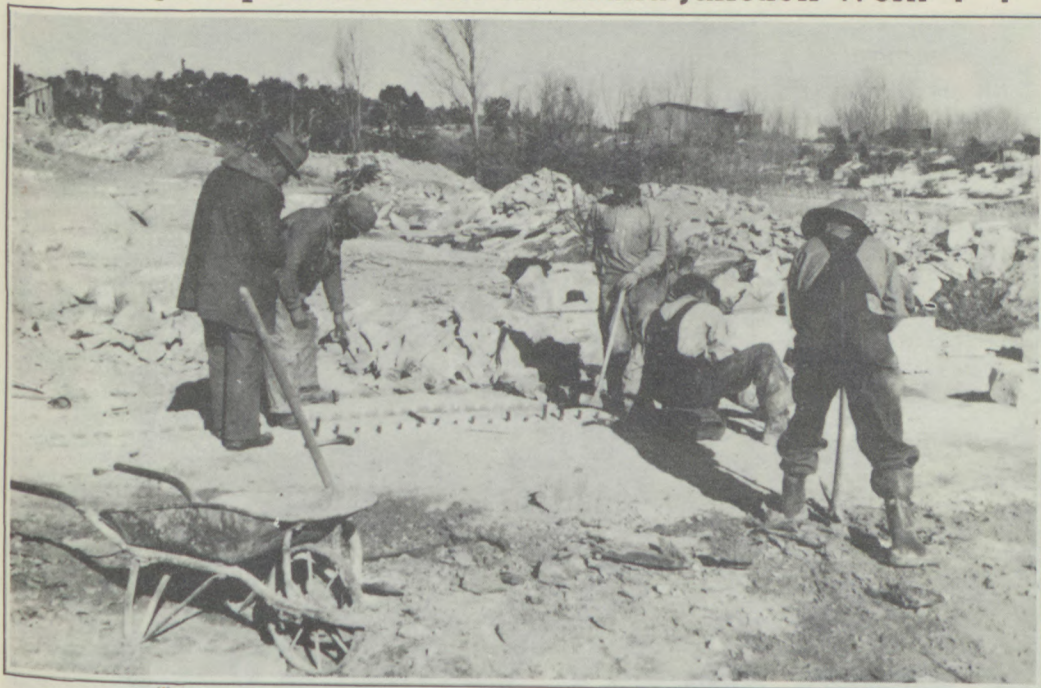
Using sledge hammers and chisels, Grand Junction Works Progress Administration employees quarry stone used in the construction of public buildings in Lincoln Park, largest municipal recreational spot in that city.
