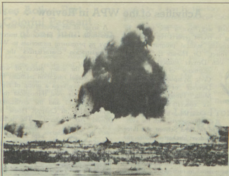
Dynamite was used in blasting loose hardened adobe which blocked the new flood control channel of the Fountain river at Pueblo. After the adobe was pulverized the river current carried away the dirt, saving excavation costs.
