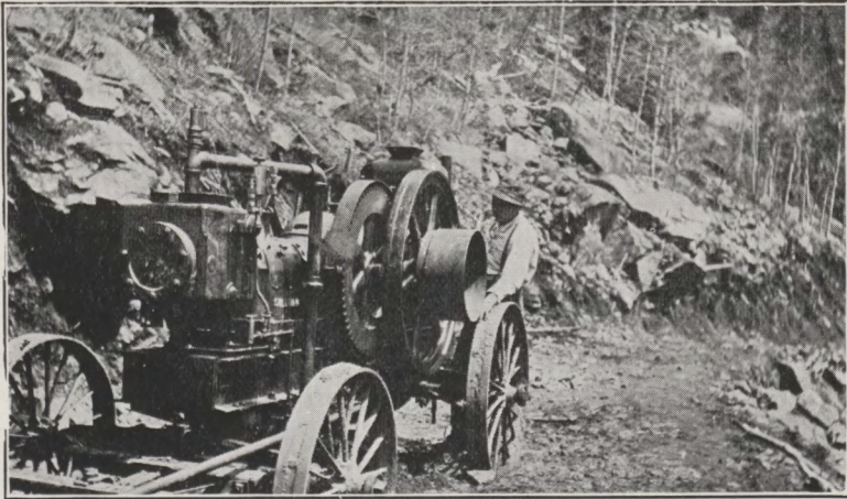
PORTABLE AIR COMPRESSOR AND DRILLING WORK ON FALL RIVER ROAD, LARIMER COUNTY (CONVICT WORK) STATE PRIMARY ROAD NO. 51
