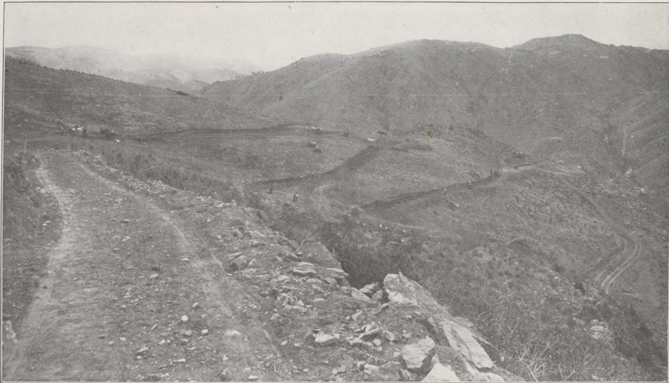
THE THREE HAIRPINS, UNDER CONSTRUCTION
