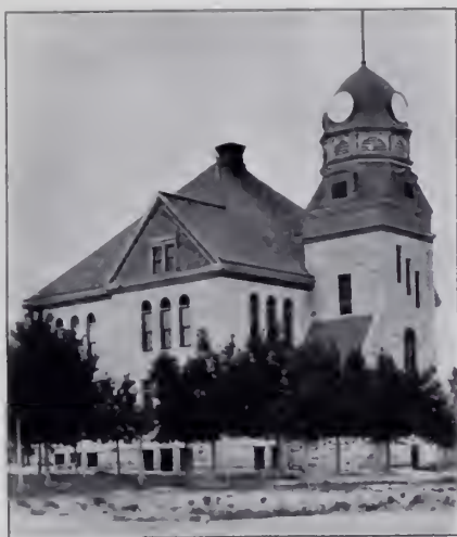
HIGH SCHOOL, LA JUNTA, OTERO COUNTY, COLO.
