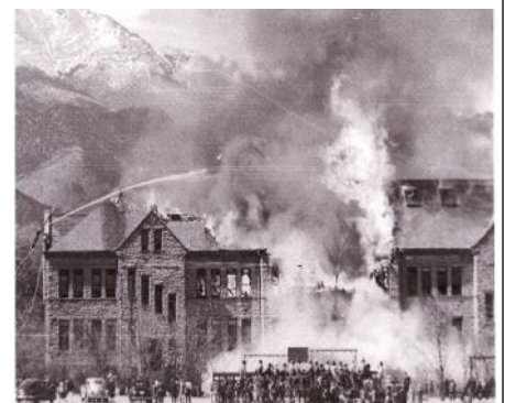
Old School Building burns while firemen use water in hoses. Pikes Peak in the background
