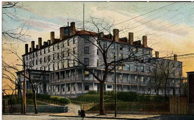
Perkins School, South Boston. 1838 hotel building used from 1839-1912
