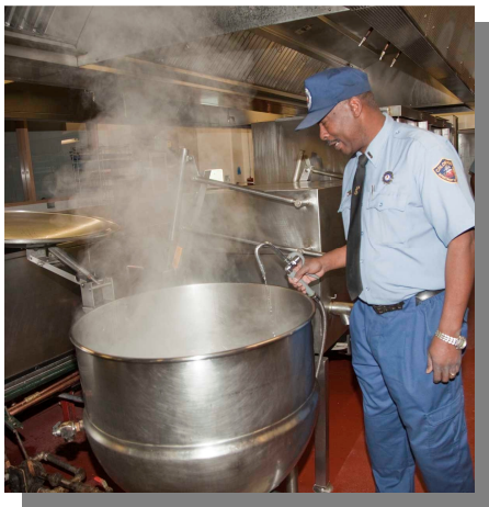
Correctional Support Trades Supervisor II
