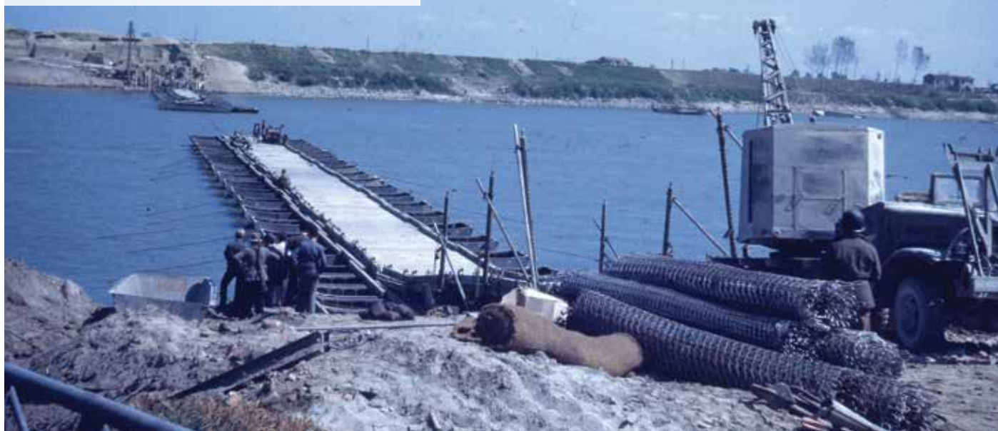
A pontoon bridge under construction which will carry the division across the Po River. History Colorado, 2020.44.51
