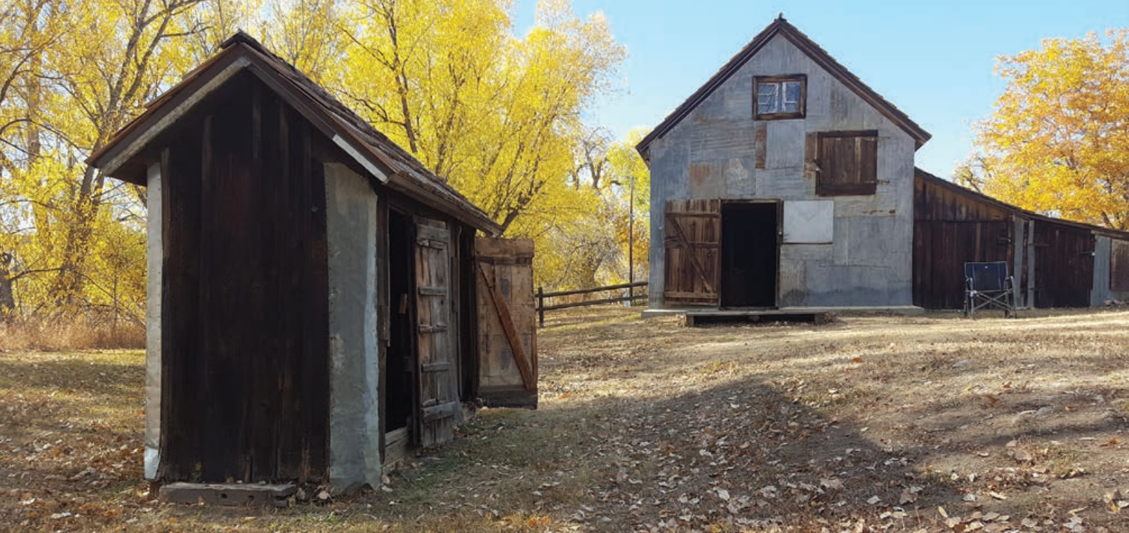
Barn and outhouse at Grasso Park, November 2021. Photo by Lindsey Flewelling.
